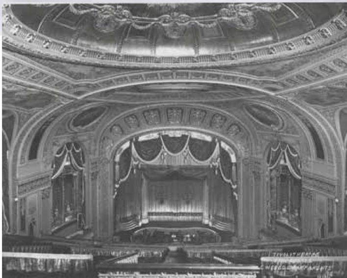
Top: Tivoli Theatre exterior; Bottom: Tivoli Theatre interior with oval orchestra pit
